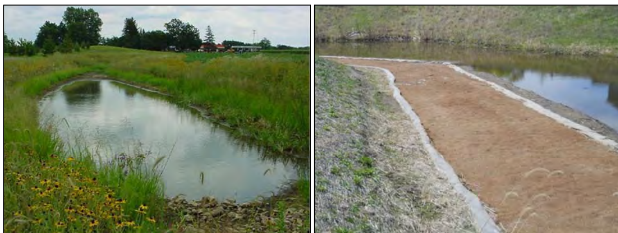
Iron-Enhanced Sand Bench, Prior Lake, Minnesota. Photographs from the Minnesota Stormwater Manual, courtesy of Mr. Ross Bintner.
