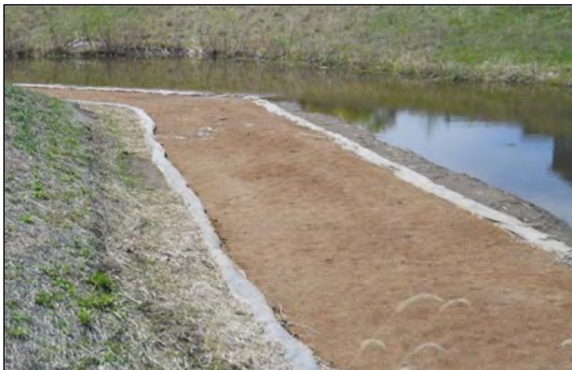
Iron-Enhanced Sand Bench, Prior Lake, Minnesota. Photograph from the Minnesota Stormwater Manual, courtesy of Mr. Ross Bintner.
